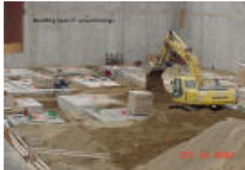
Examples of spread footings for residences and buildings.
