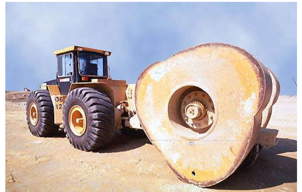
Impact Roller to Compact the Ground
