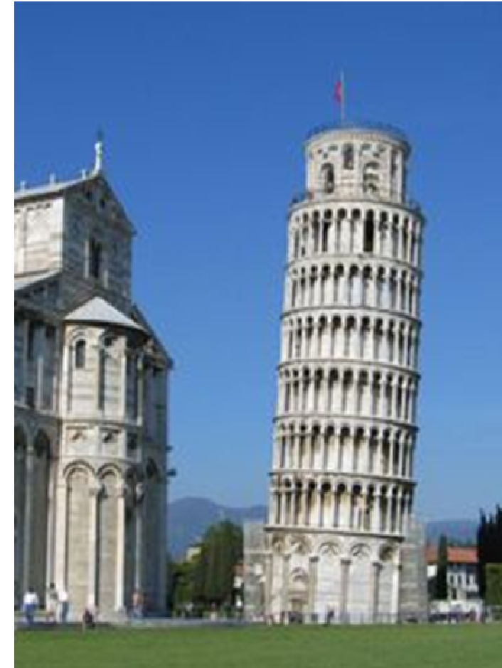
Leaning Tower of Pisa Differential Settlement
