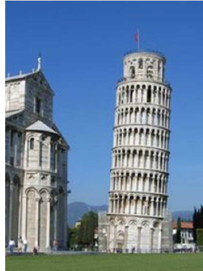
Leaning Tower of Pisa Differential Settlement
