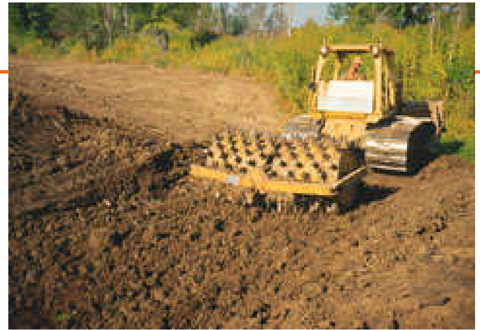
Sheepsfoot Roller to Compact Clay Soils
