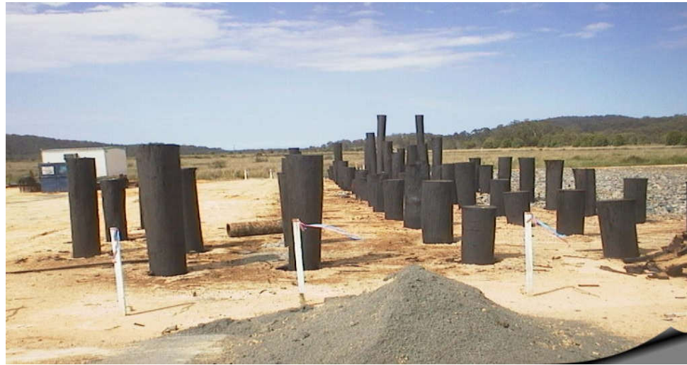
Driven timber piles, Pacific Highway
