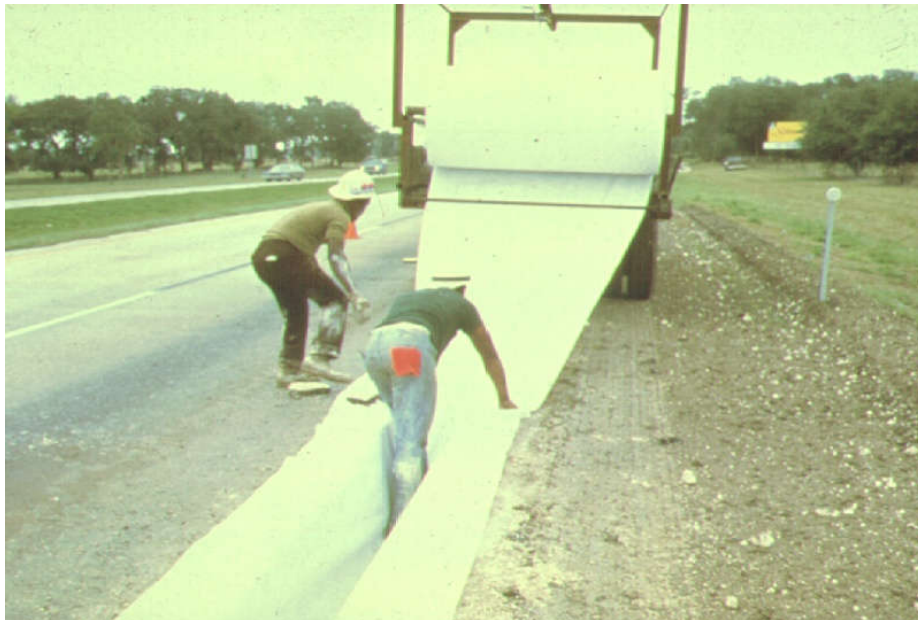
(GT Filter in Excavated Trench)
