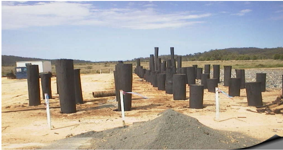
Driven timber piles, Pacific Highway
