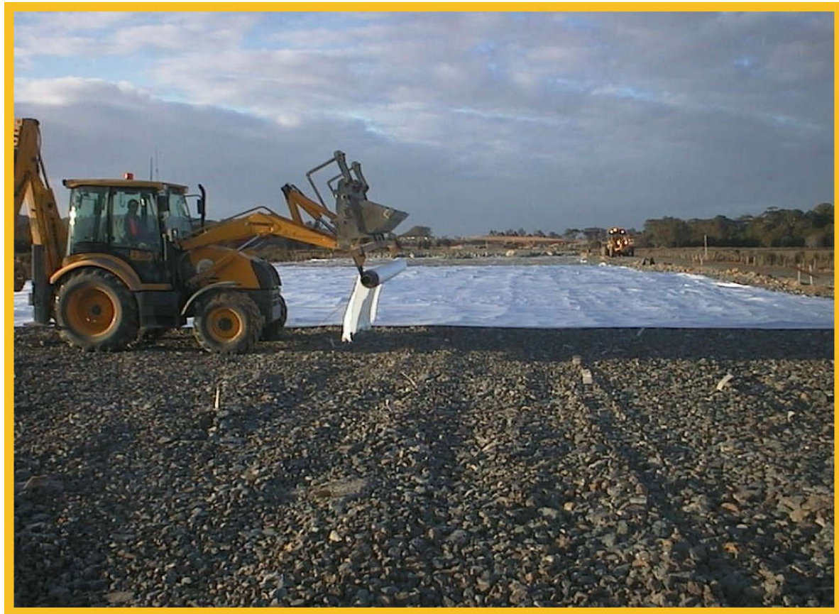
Geofabrics used on Pacific Highway
