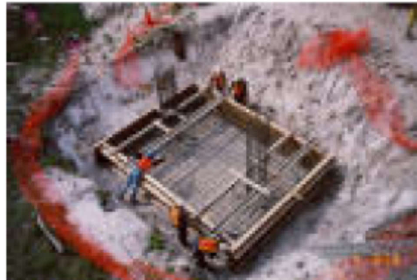
Examples of spread footings for residences and buildings.
