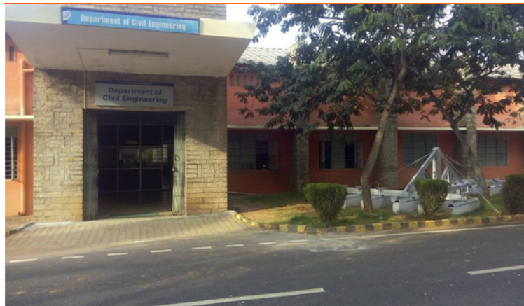
Fig 6: Department of Civil Engineering
