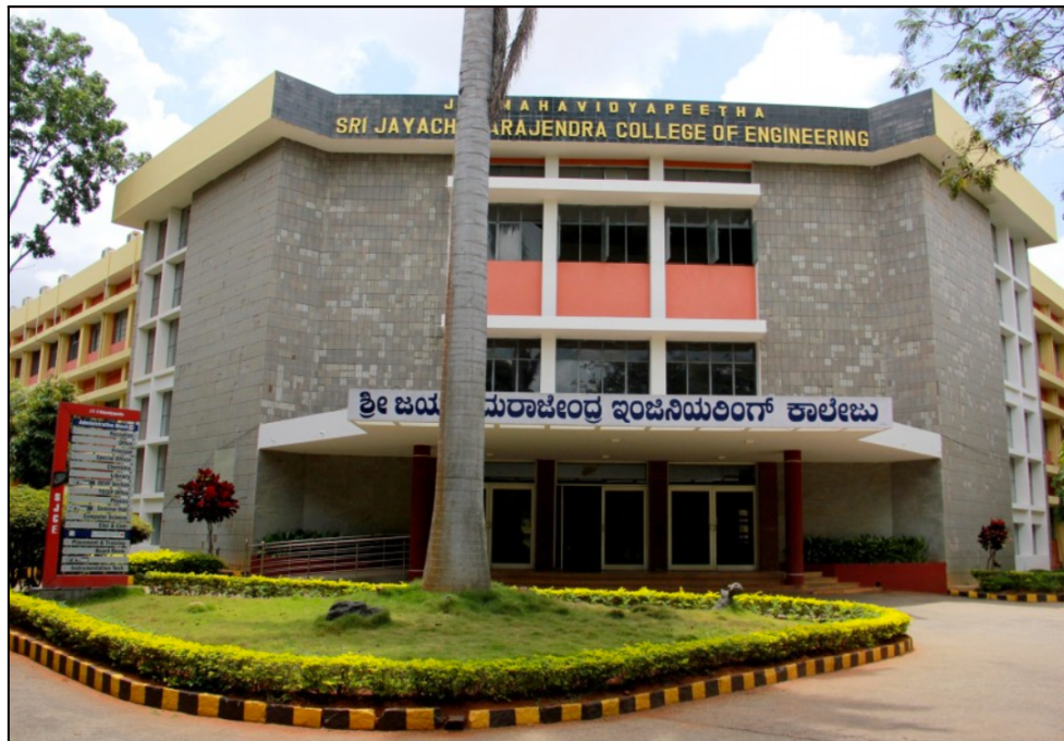
Fig 1: Administrative block of SJCE
